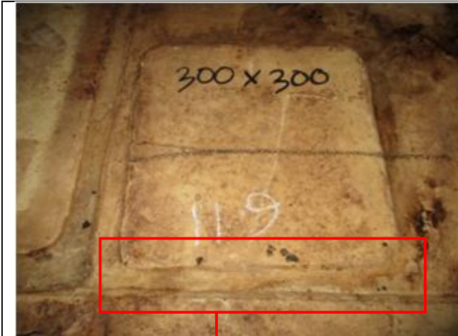
Bottom Plate - Plate number: 3-1 (300x300mm)
