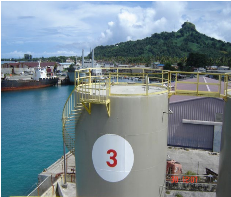
Tank Roof 1 - this picture was taken in 2010
