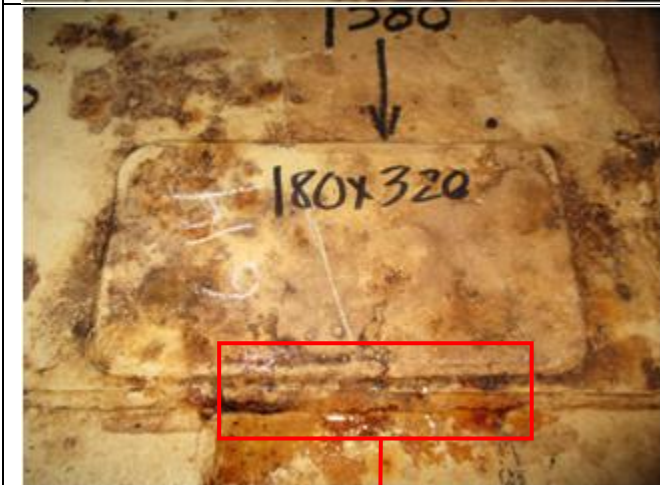
Bottom Plate - Plate number: 4-2 (180x320mm)
