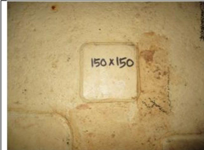
Bottom Plate - Plate number: 3-3 (150x150mm)
