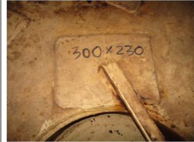
Bottom Plate - Plate number: 3-2 (300x230mm)
