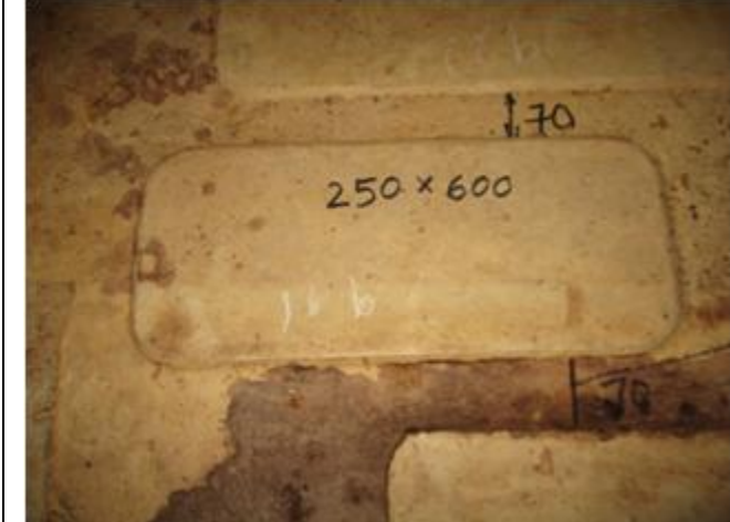
Bottom Plate - Plate number: 3-2 (250x600mm)
