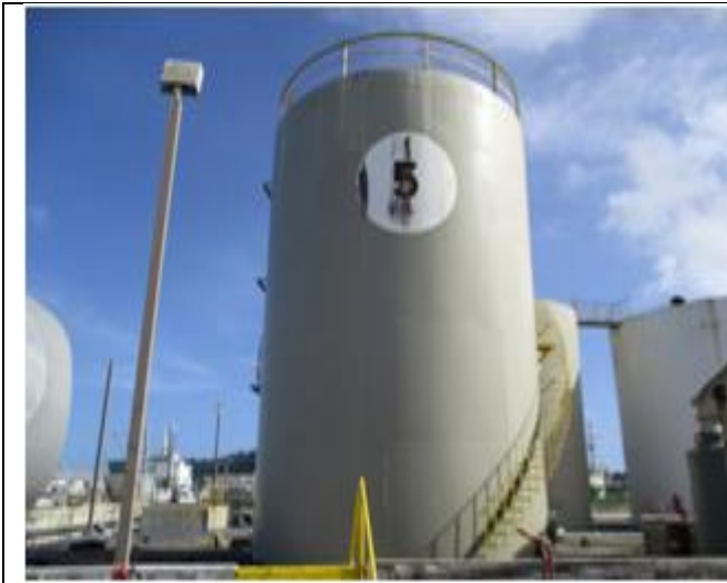
General View of Tank T5
