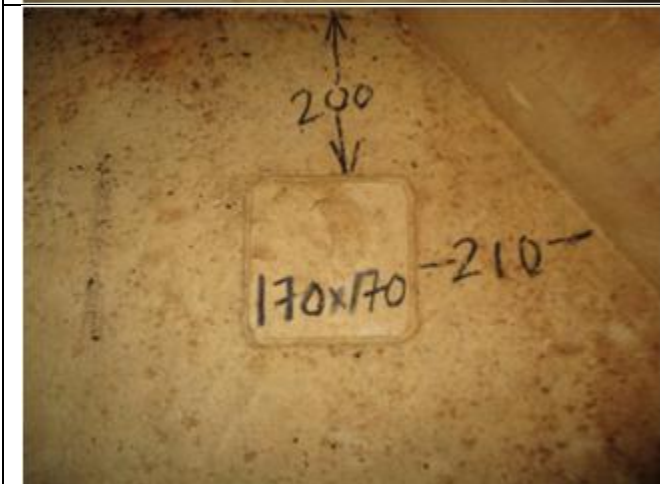
Bottom Plate - Plate number: 4-1 (170x170mm)
