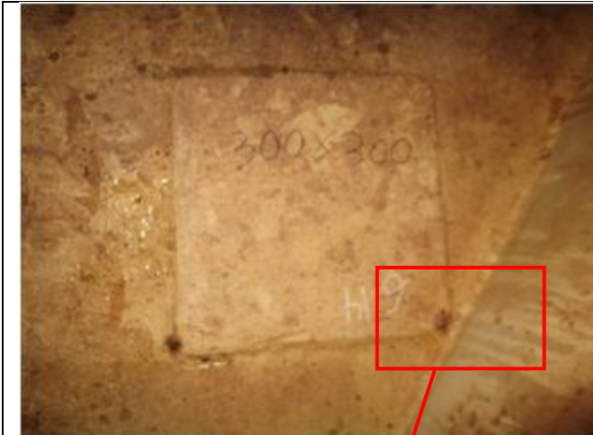
Bottom Plate - Plate number: 2-1 (300x300mm)
